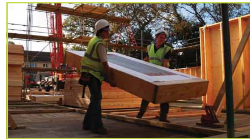
Timber frame construction underway at Shortland House.
