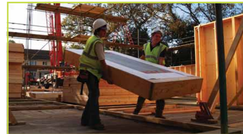
Timber frame construction underway at Shortland House.
