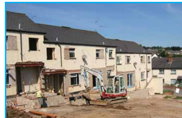
Improvement work at Foxhayes
