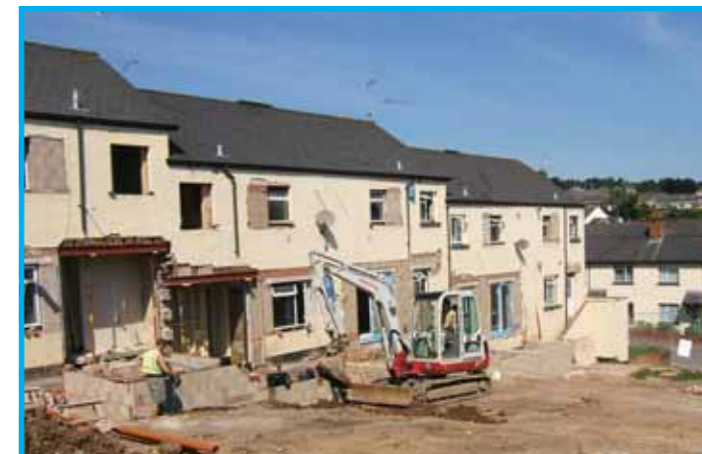
Improvement work at Foxhayes
